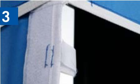
Adjoining walls can be sealed together using Velcro along sides
